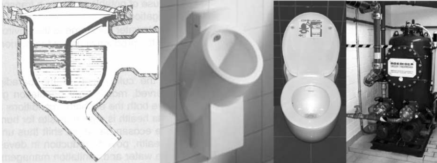
Figure 2 Siphon for waterless urinals invented by Beets, 1885: Oil forms a layer on top of the urine and stops smells (left, Lange, 2002), waterless urinal of GTZ Headquarters (middle, Keramag) and vacuum toilet and pumping station of KfW Building (right, GTZ project data-sheets 2006)
